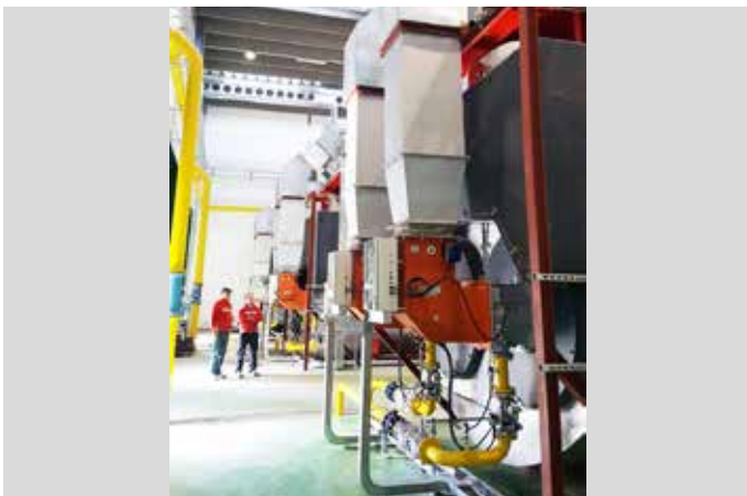
DISTRICT HEATING Burner models: No.6 IB 1200 G ME LX - electronic modulation - Low NO x combustion head - O 2 control
