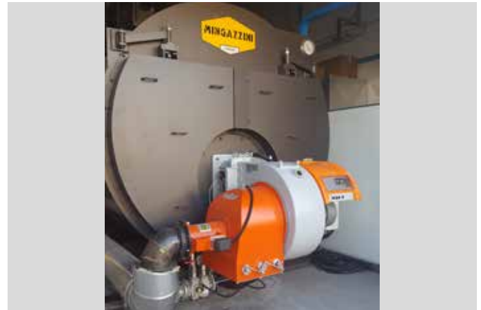
PAPER MILLS - SPECIAL PROJECT Burner model: TBG 1100 ME V O2 FGR - O 2 control, inverter and flue gas recirculation NO x <80mg/kWh
